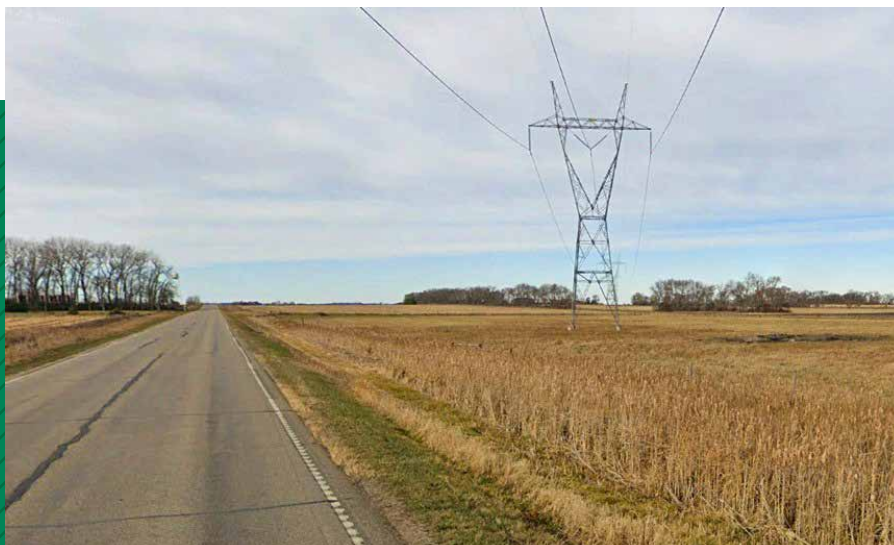
The Leland Olds Station-to-Watertown 345-kilovolt transmission line crosses roughly a mile and a half of the Lake Traverse Indian Reservation.
